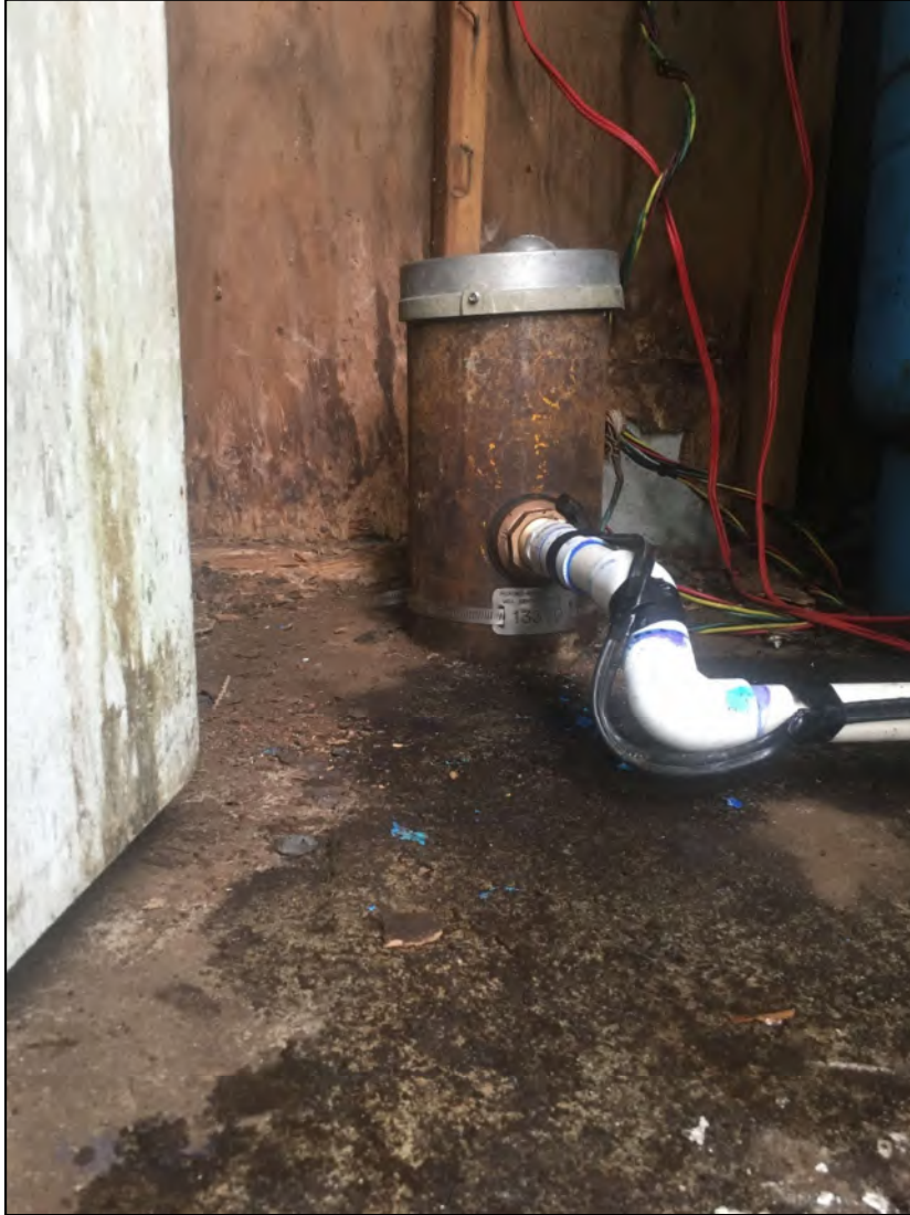
Photo C1 & C2: (LEFT) Looking west, inside the pump house of Well 13370 (Pumping Well) at the stick-up, ID plate number and well distribution piping (Photo C1). (RIGHT) Looking west, inside the pump house of Well 13370 at the distribution piping going past the flow control valve and to the flow meter (Photo C2).
